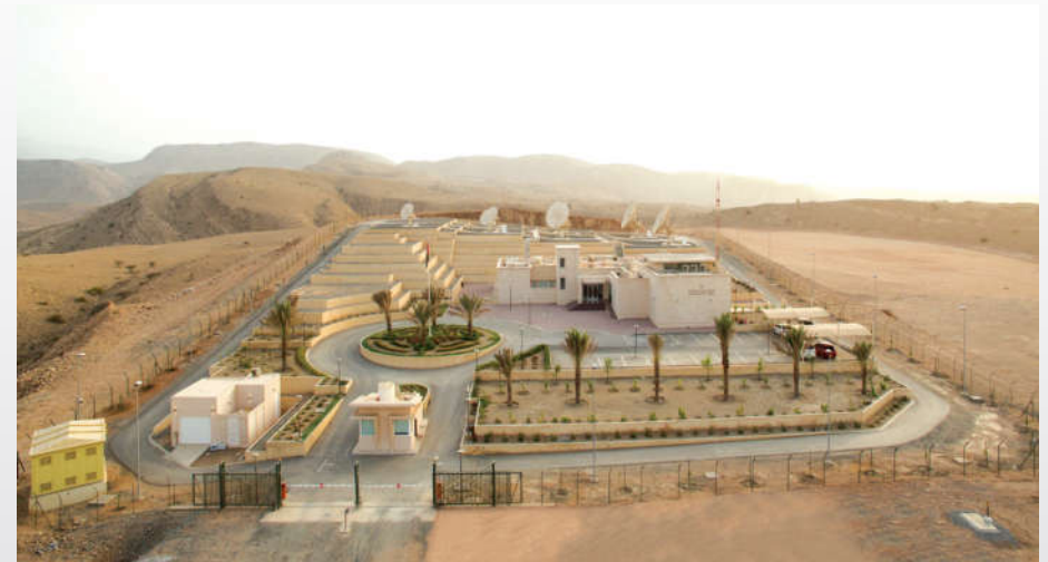
Figure 5: Aerial Photo of the Station
