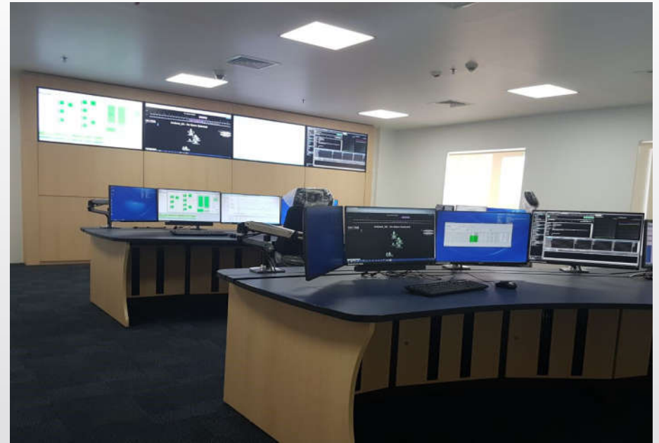
Figure 10 B: Back-up Center (TRA Head Office)
